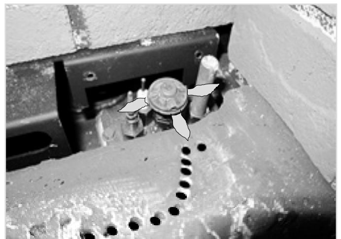
Figure 48. Use caution in placing the logs to ensure that the pilot carry-over ports are not obstructed.
