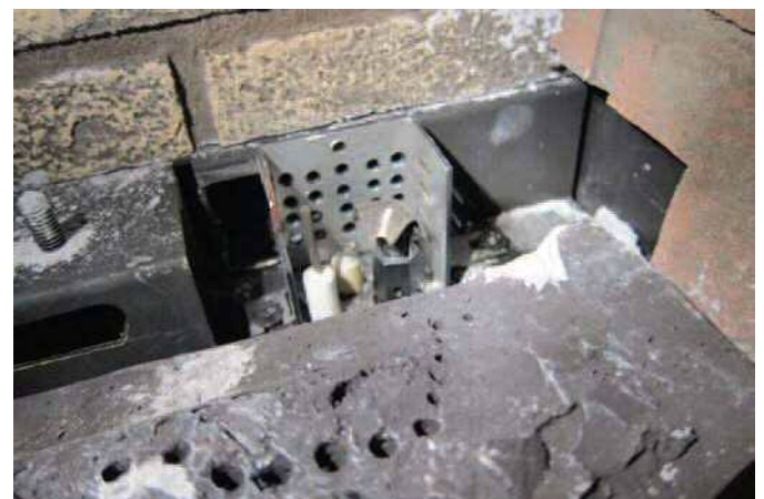
Figure 47. Use caution in placing the logs to ensure that the pilot carry-over ports are not obstructed.
