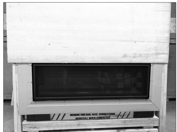
Figure 4.9, Installed Panels and Non-Combustible Material
