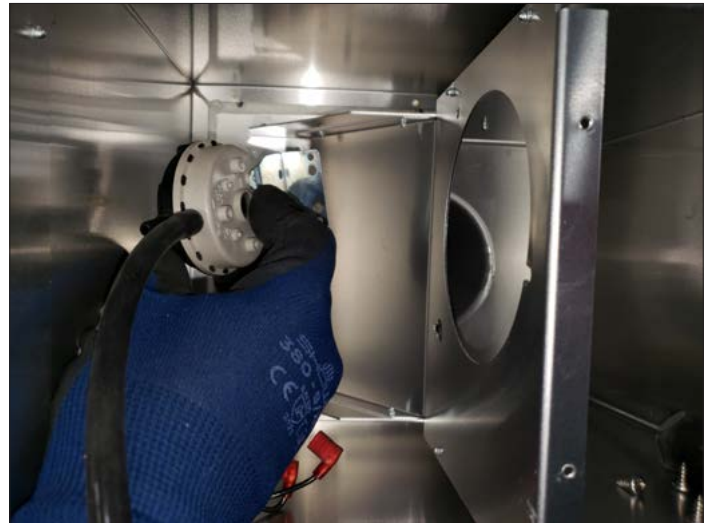
Figure 5.9, Vacuum Switch Removal
