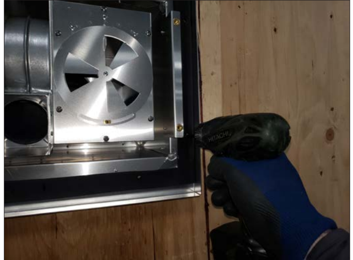
Figure 3.20, Install Cap into Wall
