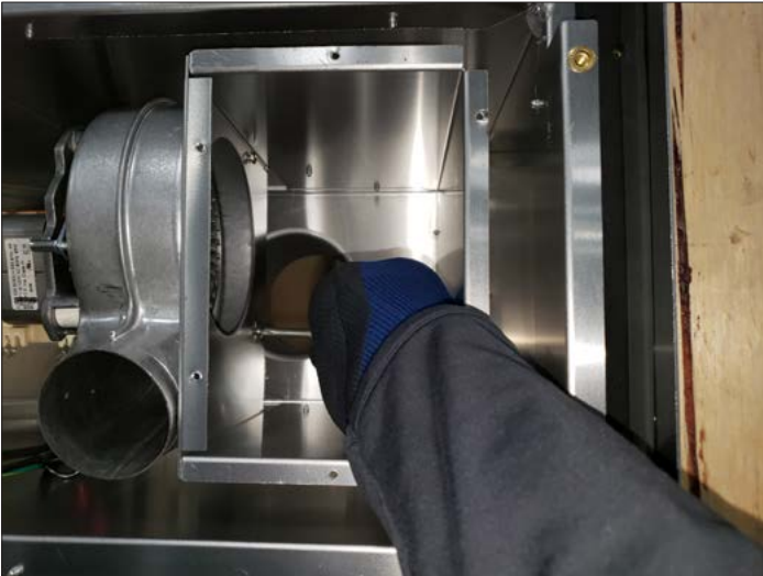
Figure 5.6, Remove (3) Screws Securing Fan Assembly
