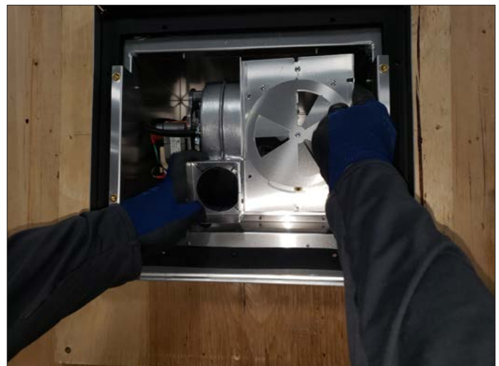
Figure 5.3, Exhaust Assembly Removal
