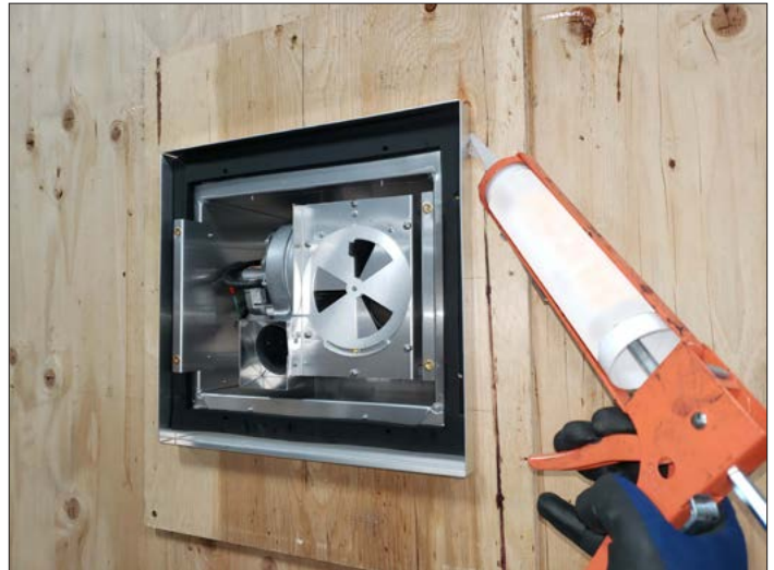
Figure 3.21, Silicone around the Cap Base
