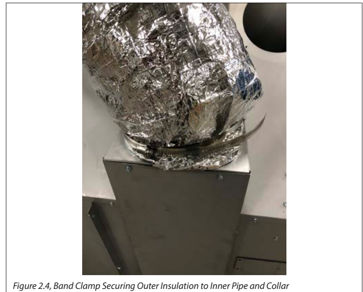
Figure 2.4, Band Clamp Securing Outer Insulation to Inner Pipe and Collar
