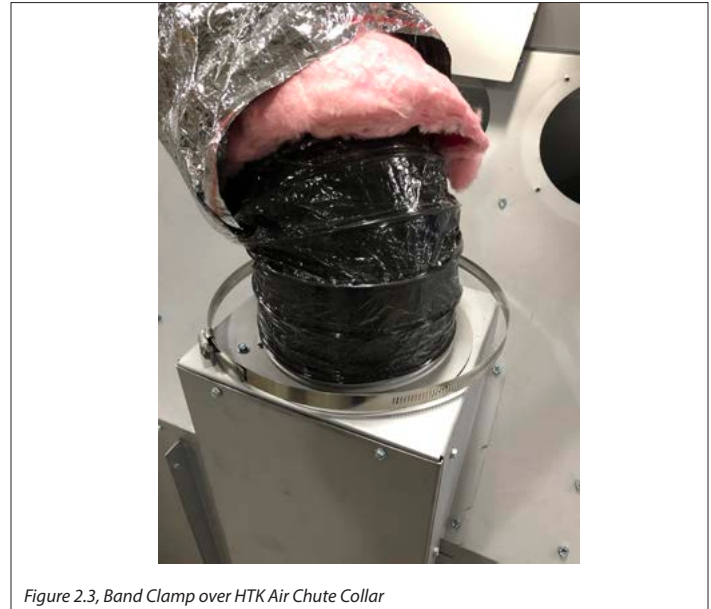
Figure 2.3, Band Clamp over HTK Air Chute Collar
