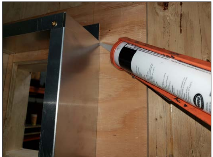
Figure 2.10, Silicone Perimeter
