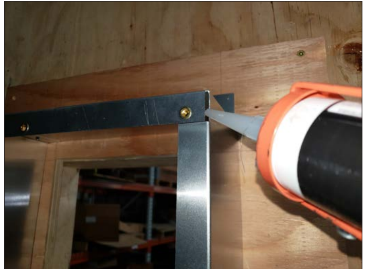
Figure 2.9, Silicone Corners
