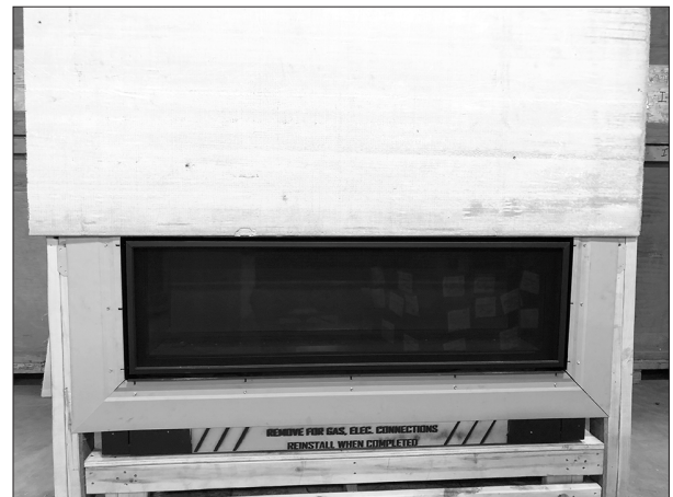
Figure 4.9, Installed Panels and Non-Combustible Material
