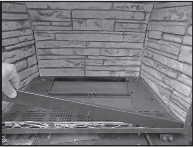
Figure 73: Covering wires with front trim piece.
