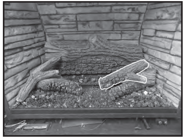
Figure 83: 5th log in place.
