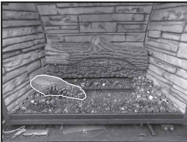
Figure 80: 2nd log in place.
