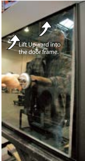
Figure 17. (Lift the door upward)
