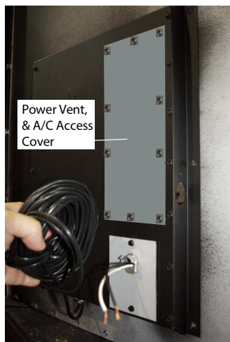
Figure 12a. Remove Exterior Access Cover.
