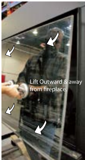
Figure 17. (Lift the door upward)
