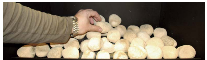
Figure 23.q Place the fourth Top faux Rock on top of the previous (2) two Rocks.
