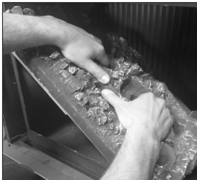
Figure 13. Burner Removal - Rotate 45 degrees
