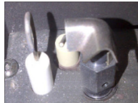
Figure 25 Proper Pilot Position
