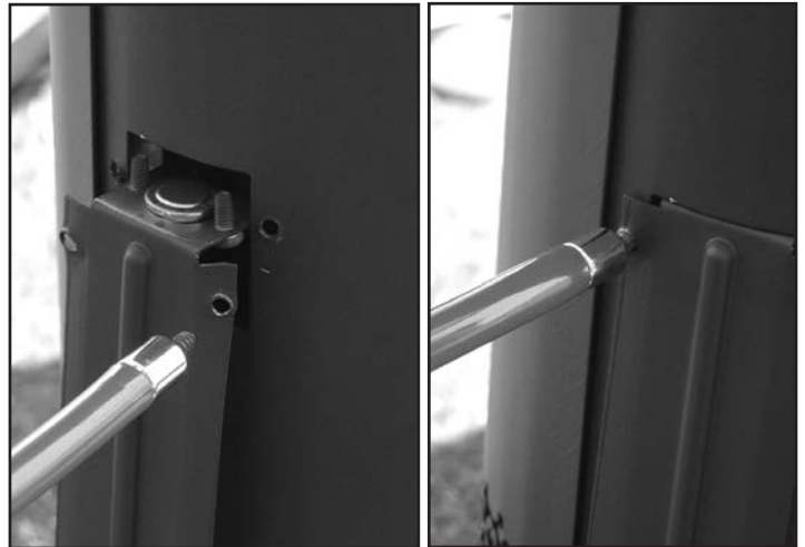
Figure 48: Spill switch installation.
