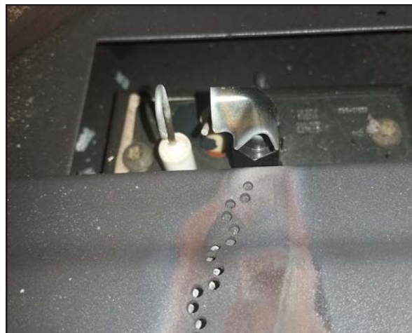
Figure 2. Correct Pilot
