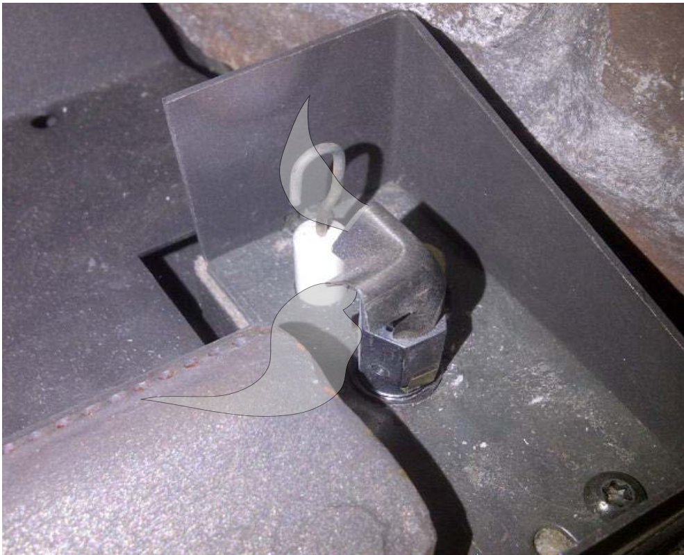
Figure 21. Correct Burner & Pilot Shield Placement
