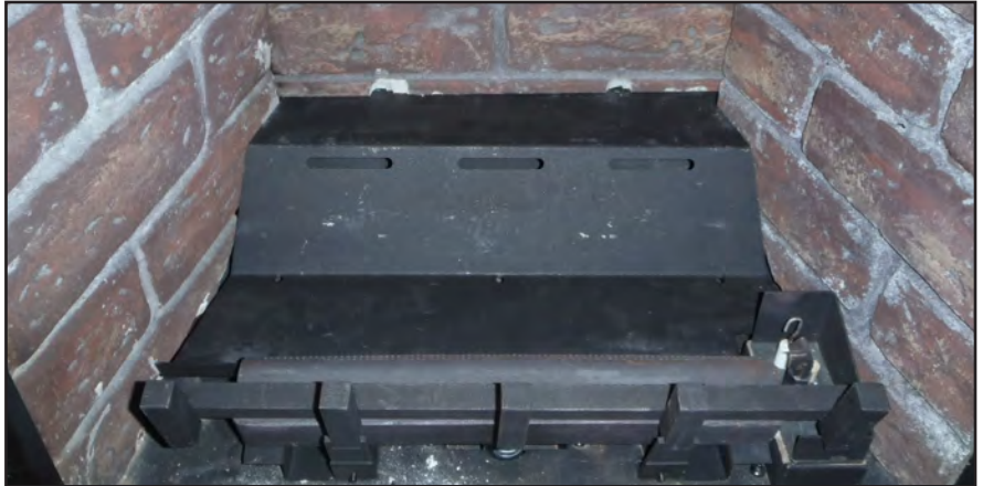
Figure 41. Empty firebox with grate and locator pins.
