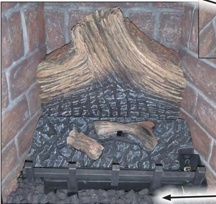
Figure 43. Coal Nuggets Installation.
