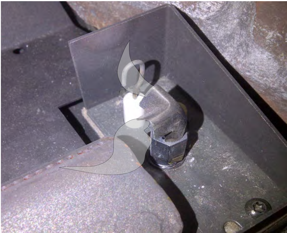
Figure 21. Correct Burner & Pilot Shield Placement
