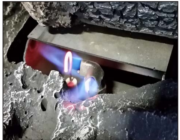
Figure 28. Correct Pilot
