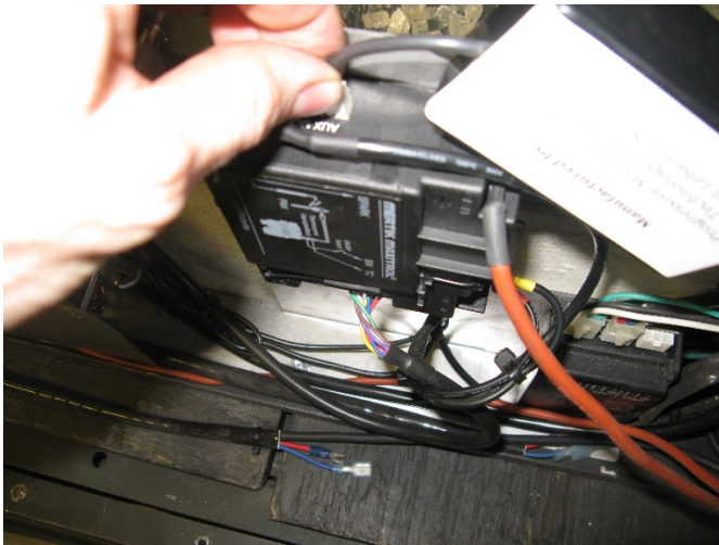
Plug in the power vent relay harness HRD-803 to the AUX port on the fireplace control.
