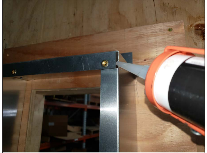
Figure 2.9, Appliquez le scellant silicone aux coins
