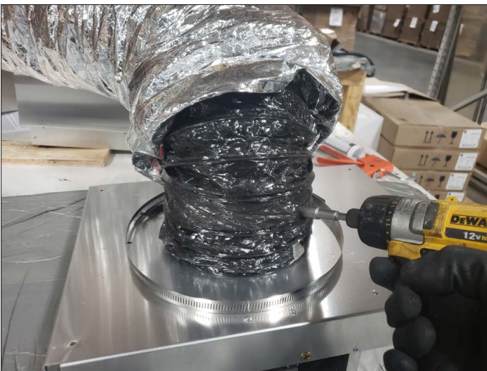
Figure 2.16, Screws in Inner Liner
