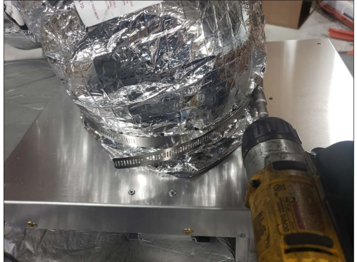
Figure 2.17, Liner Installed with Band Clamp
