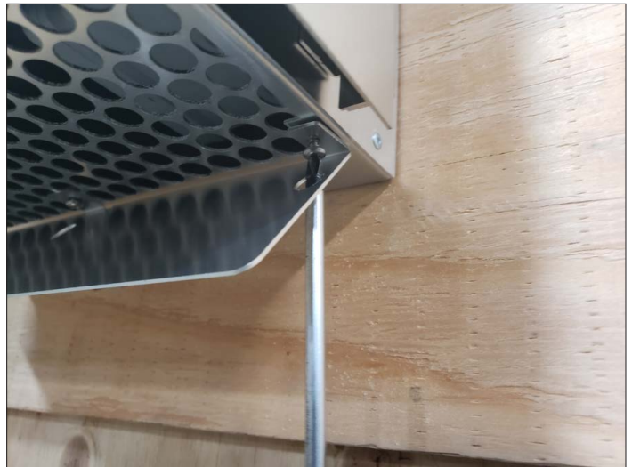
Figure 2.18, Vinyl Siding Installed
