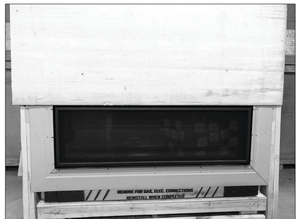
Figure 4.9, Installed Panels and Non-Combustible Material
