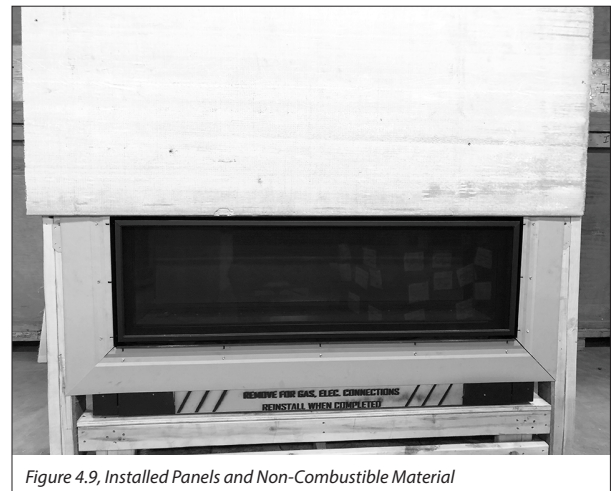
Figure 4.9, Installed Panels and Non-Combustible Material
