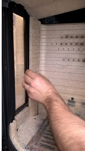
Remove the steel skamol bracket, holding the Upper baffle plate.
