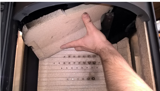
Remove the Upper baffle plate, by lowering the left side. now there is a clear path to the smoke outlet.
