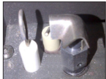
Figure 23: Proper Pilot Position
