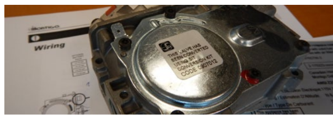
Figure 13.k Conversion label on valve
