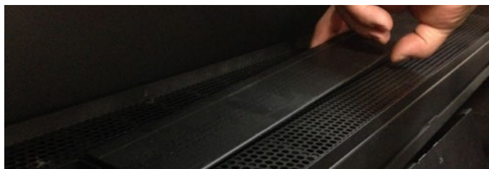
Figure 13.b Loosening the venturi
