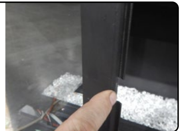
Figure 21.b Installing the door
