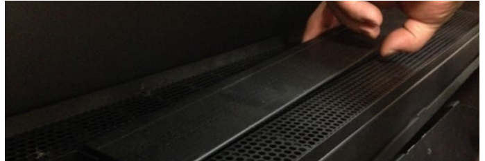
Figure 13.b Loosening the venturi
