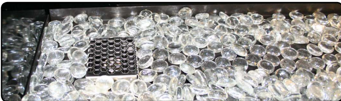
Figure 24.b Completed firestone installation
