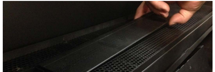
Figure 13.b Loosening the venturi
