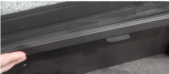
Figure 20.b Lift out the Retaining Tabs and screen
