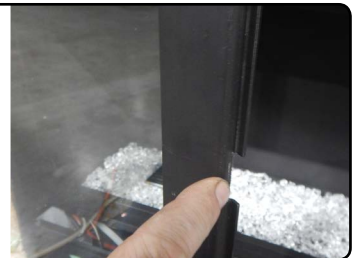
Figure 21.b Installing the door
