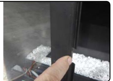
Figure 21.b Installing the door
