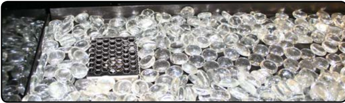
Figure 24.b Completed firestone installation
