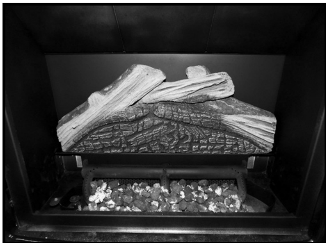
Figure 47: Number 1 log set in place.
