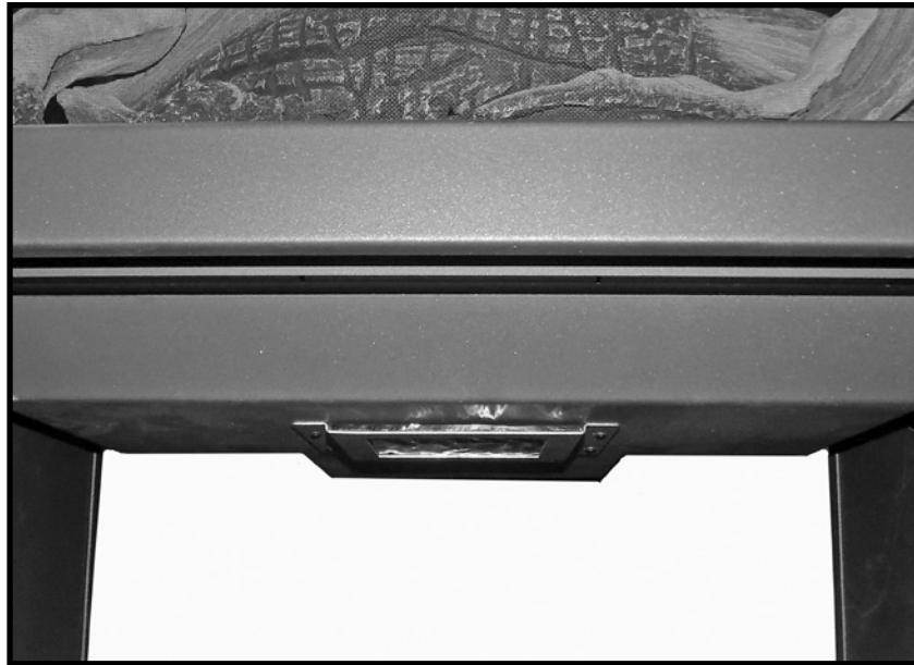
Figure 63: TN24 glass plate holder location.
