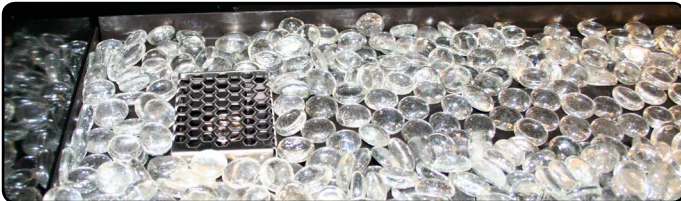
Figure 24.b Completed firestone installation
