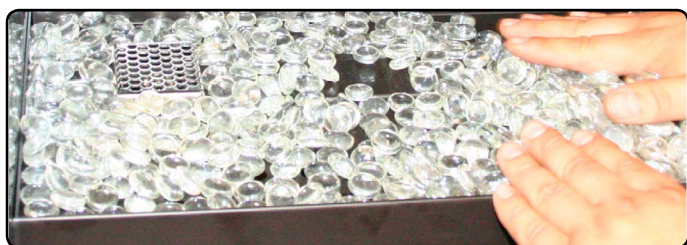
Figure 24. spreading out firestones
