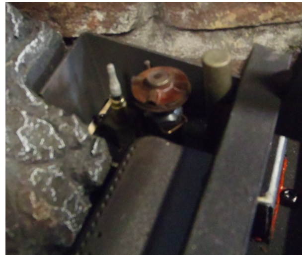
Figure 15. Pilot assembly beside the burner.
