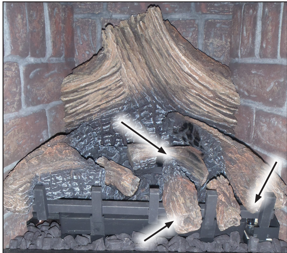
Figure 39. Fourth Stage Log Set Installation.
