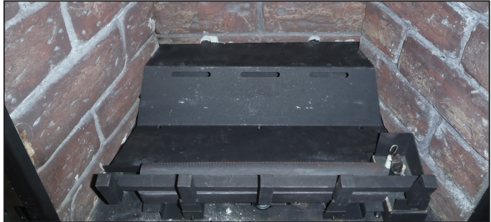
Figure 35. Empty firebox with grate and locator pins.
