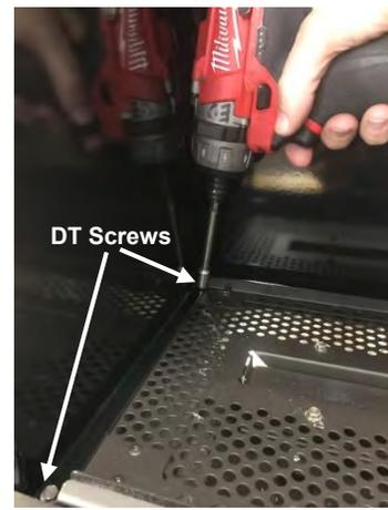
**STEP THREE:** Fasten top of panel with One DT Screw.
