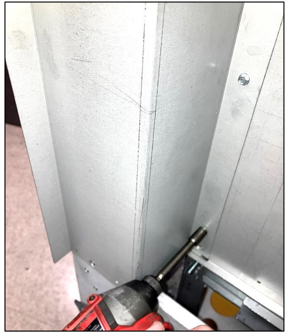
Attach Front Side Cover with DT Screws
