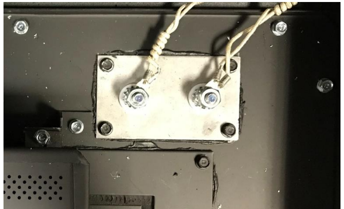
BOTH LAMP ASSEMBLIES ARE CONNECTED
