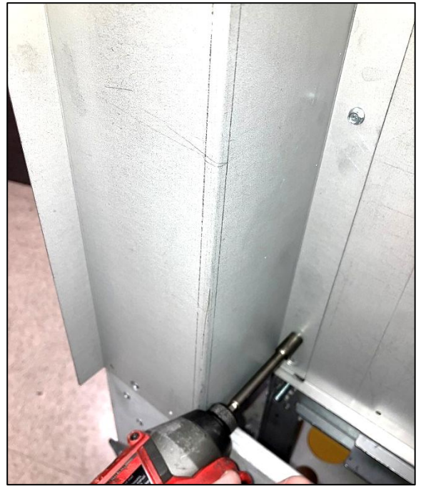
Attach Front Side Cover with DT Screws
