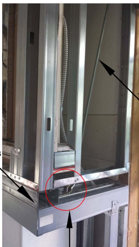
CONNECTION POINT FOR 3/4" ALL THREAD ROD TO HEADER
