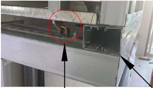
CONNECTION POINT FOR 3/4" ALL THREAD ROD TO HEADER
