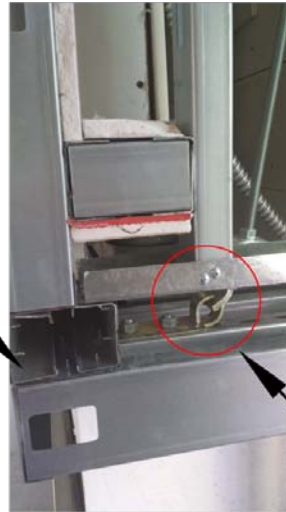
CONTINUOUS BOX HEADER SIDE VIEWS
