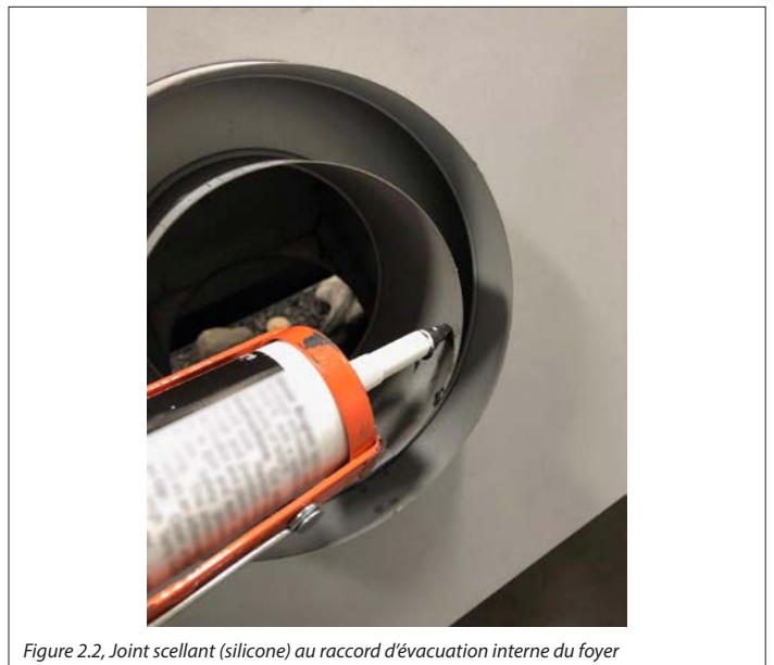
Figure 2.2, Joint scellant (silicone) au raccord d'évacuation interne du foyer
