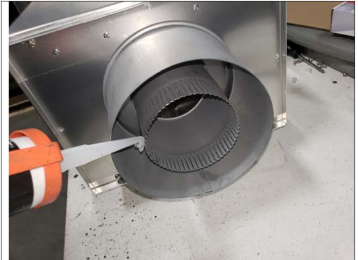
Figure 2.1, Silicone Inner Exhaust on Power Vent Assembly
