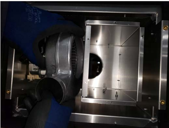
Figure 5.7, Fan Assembly Removal
