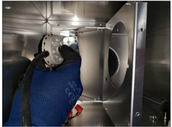
Figure 5.9, Vacuum Switch Removal
