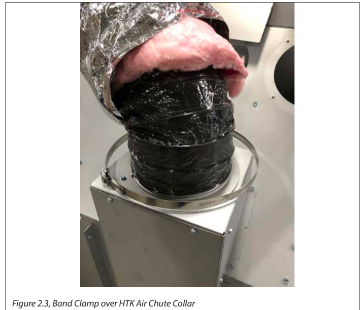
Figure 2.3, Band Clamp over HTK Air Chute Collar
