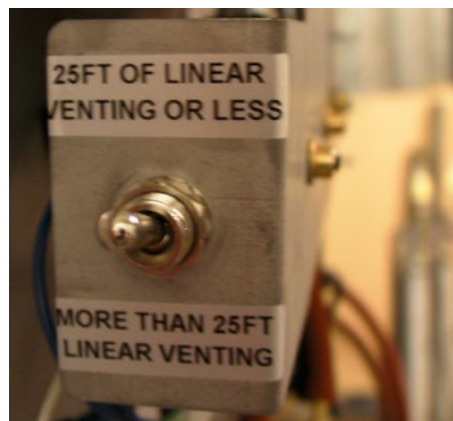
Figure 38a. Vent Selector Switch
