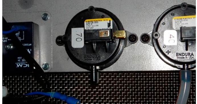
Figure 117. Disconnect grey wire.
