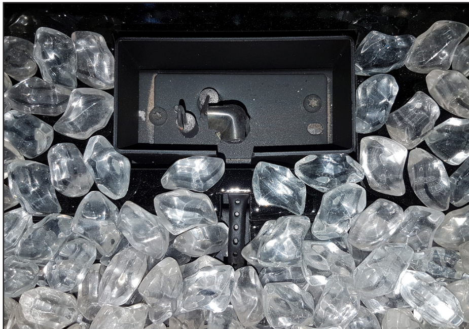
Figure 49: Correct glass media placement around pilot area
