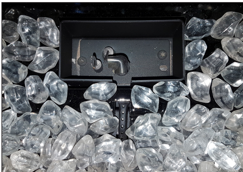
Figure 47: Correct glass media placement around pilot area
