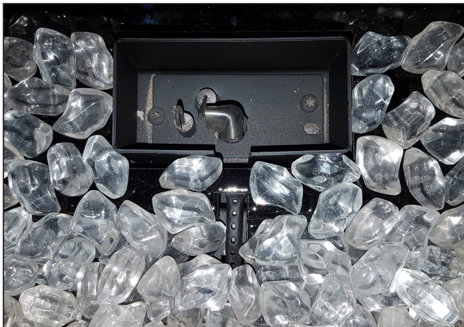
Figure 49: Correct glass media placement around pilot area
