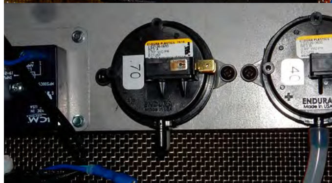
Figure 117. Disconnect grey wire.
