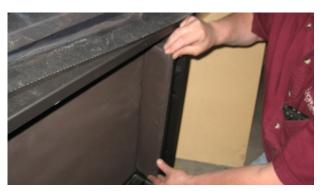
Slide one of the "keyed" side panels to the right hand side of the back contemporary panel. The tab portion to the back, beside the back contemporary panel.
