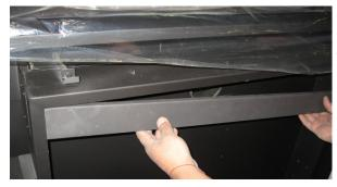
After the panels have been installed, insert the sheetmetal baffle. Angle it into the left side all the way. Lift the right side into place and center it so it rests evenly on both side panels. The glass bead material can be installed at this time (see page#26). Reinstall burner cover to complete panel installation.
