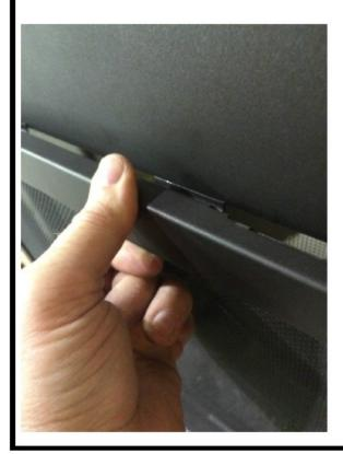
Slightly twist top part of screen frame to position top mounting tabs inside upper edge of door frame
