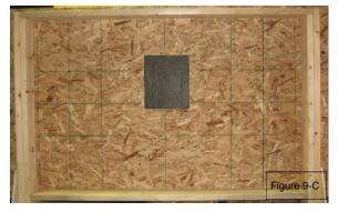
Frame hole out opening and cut out hole for the termination and thimble as shown in figure 9-A,B.
