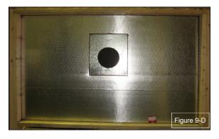
When installing in an exterior wall you must include the exterior wall insulation and termination kit. Place insulation board with the foil facing in to the room as shown in figure 9-C
