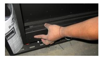
**Remove burner cover** and place to the side to be re-installed at the end.
