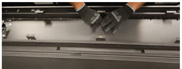
Figure 12.g Removing metal plate
