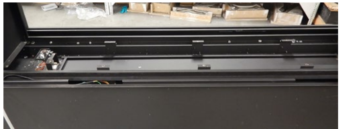
Figure 12.e Removing the Burner
