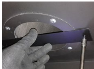
Figure 8.b.c Restrictor plate Installation
