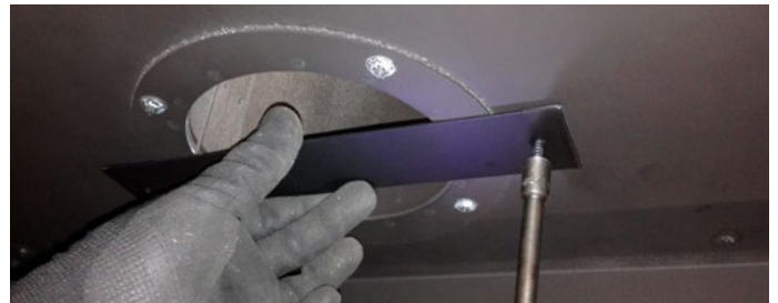
Figure 8.b.c Restrictor plate Installation
