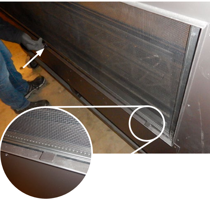
Figure 20. Locate the three tabs at the base of the screen
