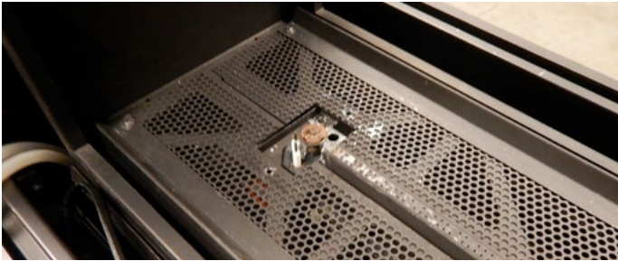
Figure 12. Removal of the pilot cover
