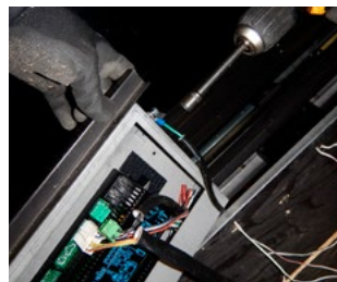
Figure 24.b Remove existing basic board
