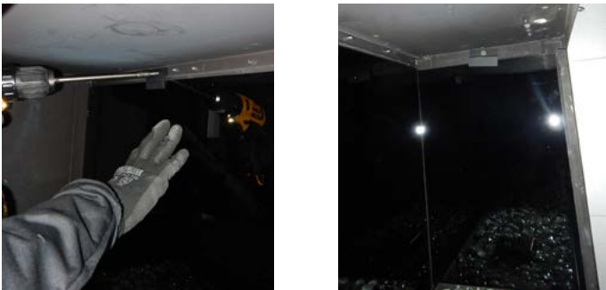
Figure 26.c Secure panel
