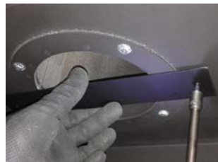
Figure 8.b.c Restrictor plate Installation
