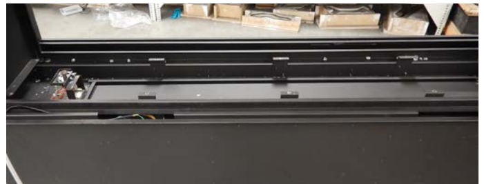
Figure 12.e Removing the Burner
