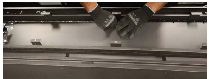
Figure 12.g Removing metal plate
