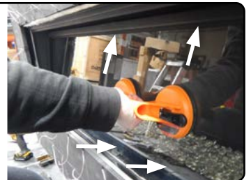
Figure 21.b Installing the door
