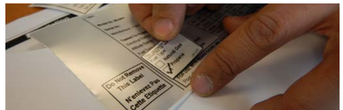
Figure 13.j Conversion label on rating plate label
