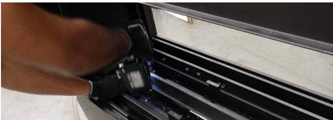
Figure 12.d Removing the Burner screws
