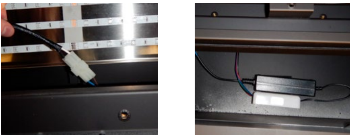
Figure 25.c. Power LED receiver
