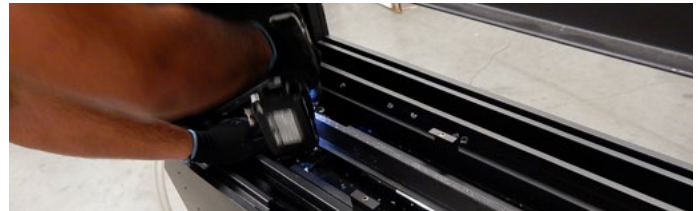
Figure 13. Removal of burner strip
