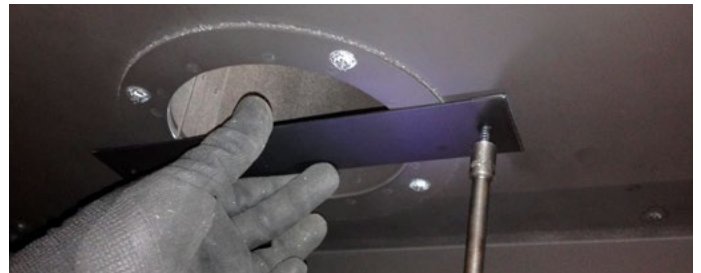
Figure 8.b.c Restrictor plate Installation
